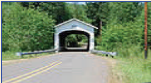
Wendling Bridge, Lane County
