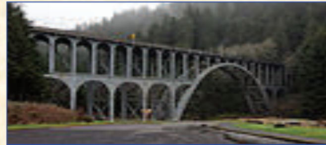
Cape Creek Bridge, Lane County
