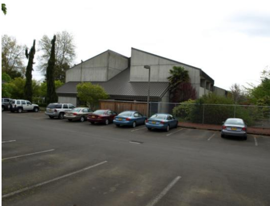
Administration – west side
