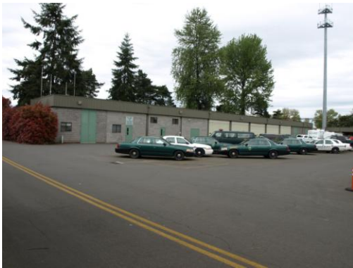
Building H (1) H.P. 2 ton
